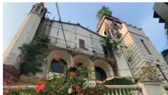
Gambar 3. Keadaan existing Hotel des Galeries
