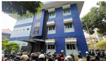
Gambar 5. Kondisi Aktual Tampak Samping FPIK B UNDIP
