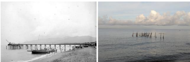
Figure 10. Ampenan Pier when it was still operational (left) and the remains of the pier's pillar structure (right).
